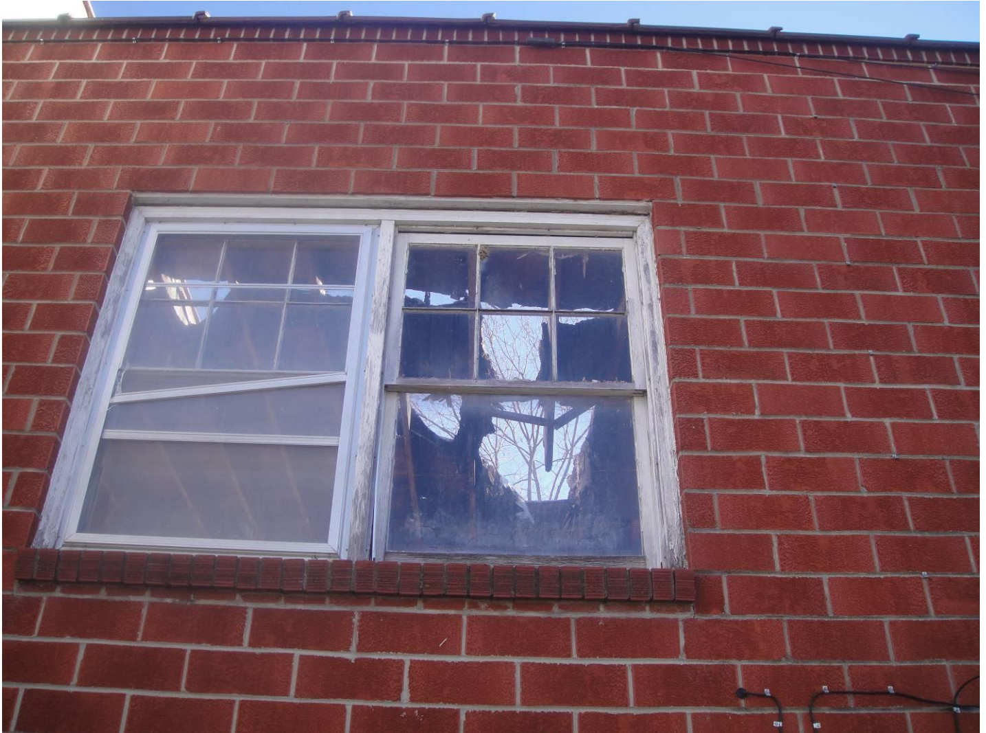
Photo 22 – View of collapsed ceiling/roof of 110 W. Main Street. View through second floor window on west side.
